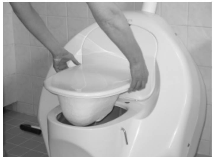
1. The seat-bowl may be lifted from its place for cleaning.
